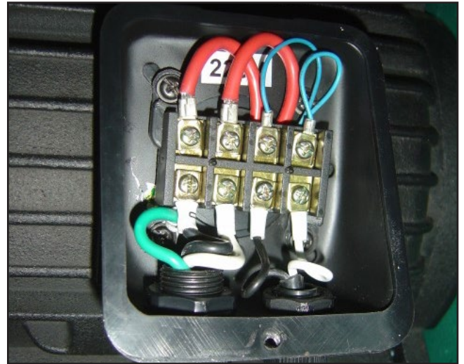
Figure 90. Motor wiring.
