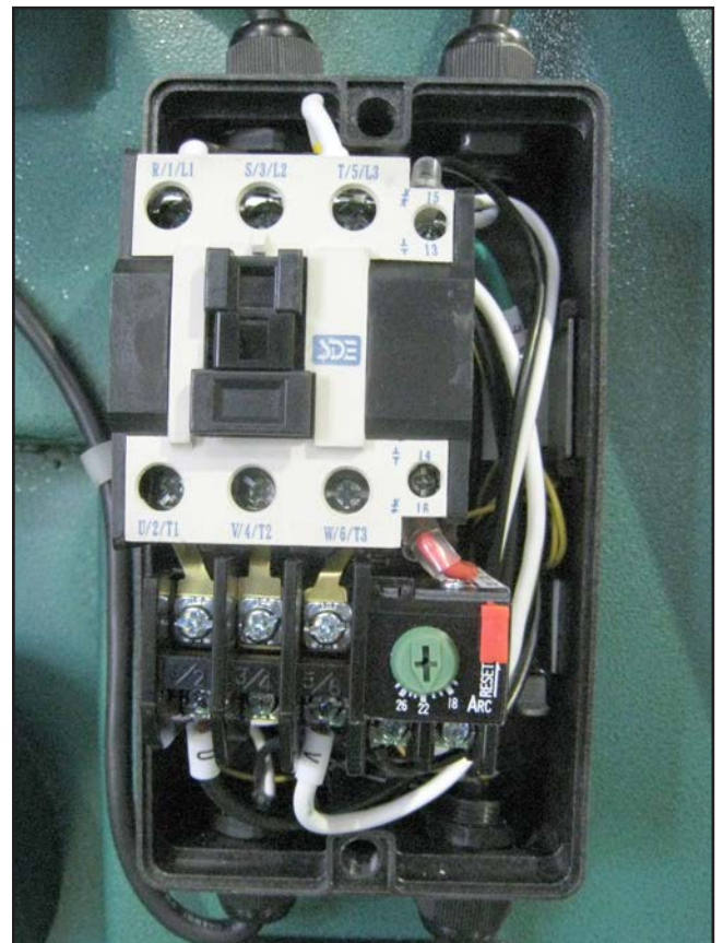
Figure 86. G0636X magnetic switch.
